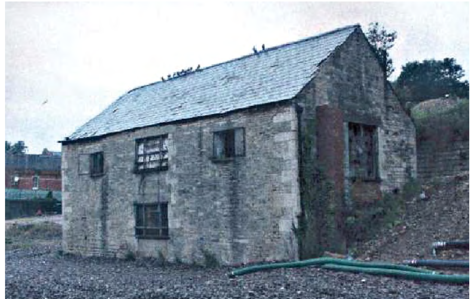
VIEW 2 : WHARF WAREHOUSE
