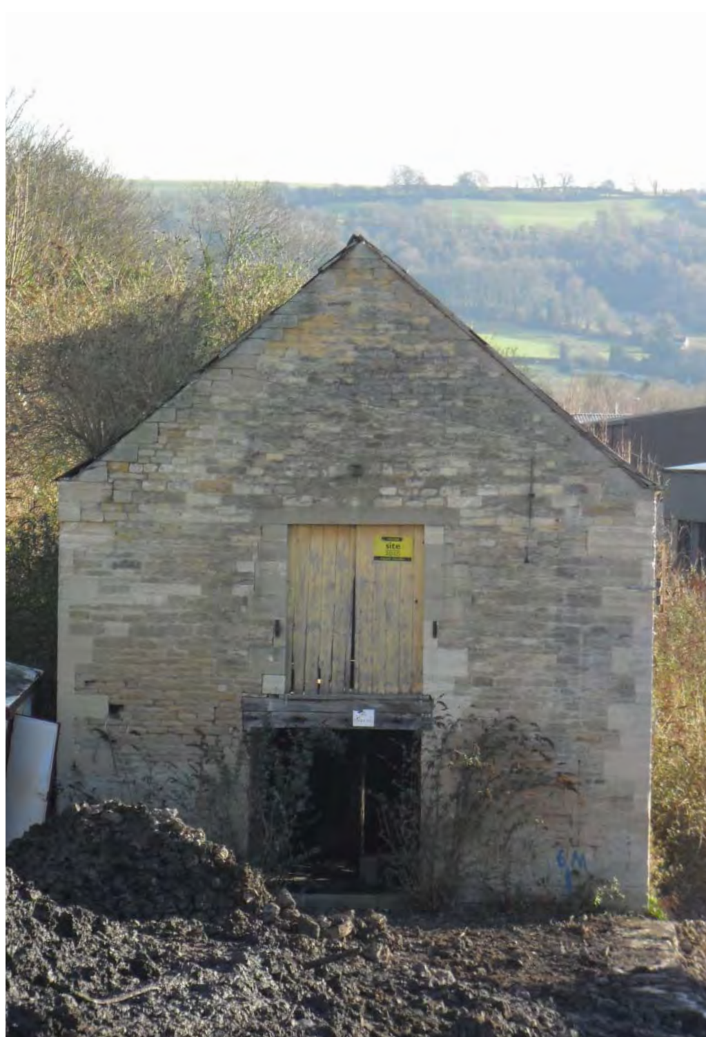
VIEW 1 : WHARF WAREHOUSE
