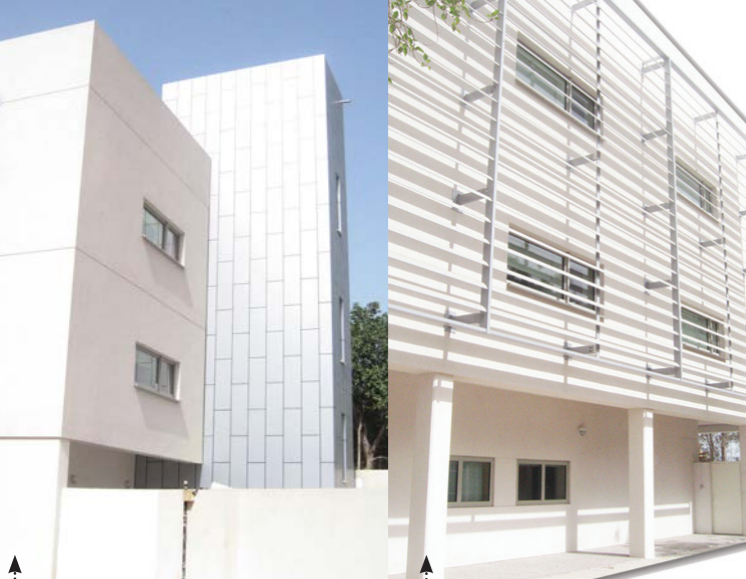
British Embassy: Abu Dhabi The project was completed in two stages: the first stage being the creation of a 390m 2 single storey secure building, the second stage was to create a further 590m 2 of accommodation of two floors above the existing building.
