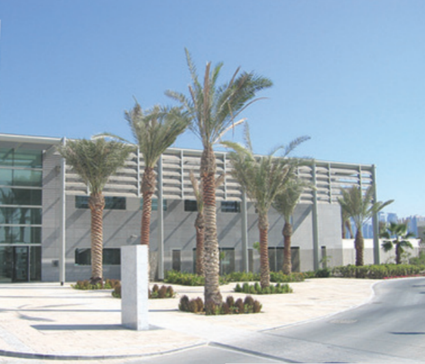
British Embassy Bahrain The building was conceived as two separate elements crossing at right angles with clerestory windows running along the length, providing light at high levels through the building. Brise soleil shading protects the building from glare and provides a comfortable working environment to the office space and public waiting area.
